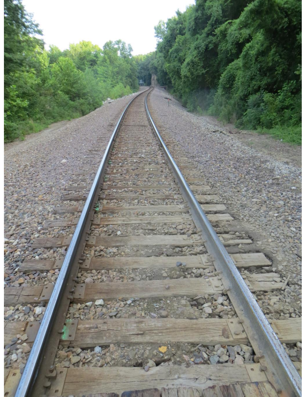
Down the tracks to the south...
